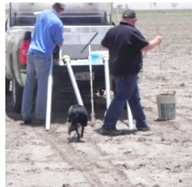
Moisture probe installation
