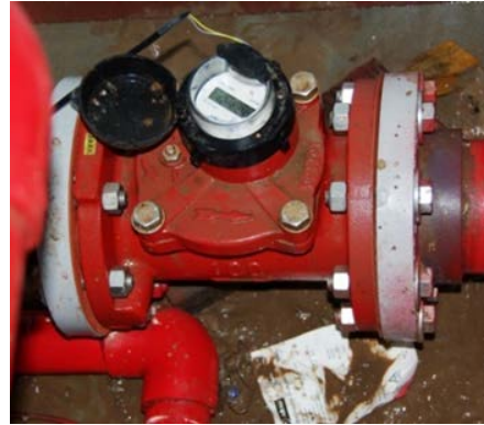
Meter on SDI drip system
