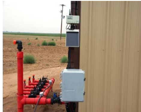
Valve bank with air relief
