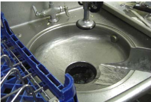
Garbage disposal and pre-rinse spray valve, Pflugerville High School, Pflugerville ISD, Pflugerville, Texas
