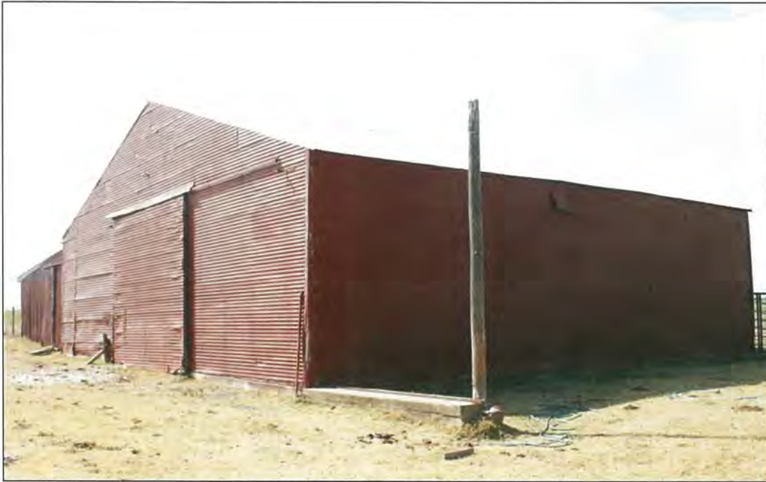
Figure 77. Resource 1c: Oblique of facade and east, looking northwest.
