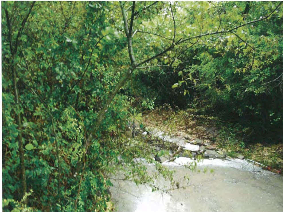
P44. Looking south (downstream) along TBC from the culvert at County Road 4945.
