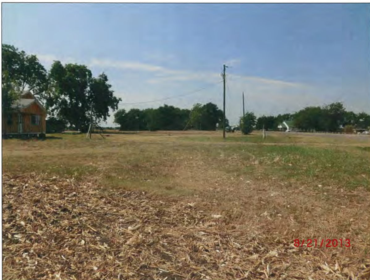
Figure 22. Structure on the northeast side of the intersection of FM 2077 and CR 3235. Note the new exterior on the structure and its foundation piers consist of modern cinder blocks.
