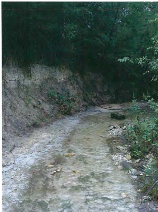
P17. Looking along steep, incised channel banks along LCT3.
