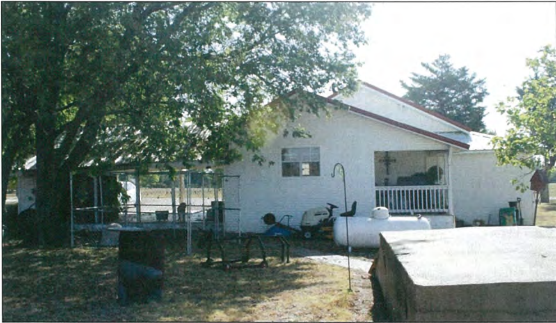
Figure 71. Resource 1a: West elevation, looking east.
