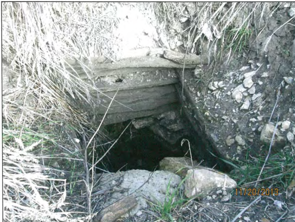
Figure 64. Close up of notched boards and dry laid limestone at 41FN174.
