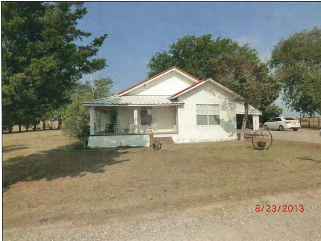
Figure 66. The house (architectural resource 1a) at 41FN175; facing east.
