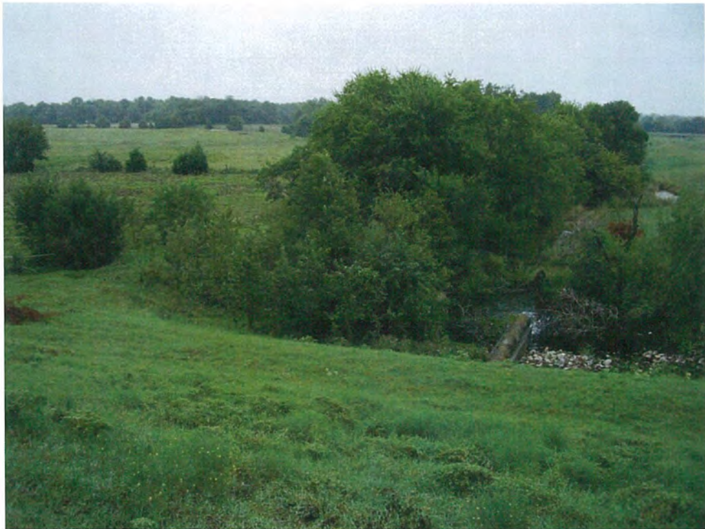
P10. Outfall for the overflow of the Lee Creek impoundment.
