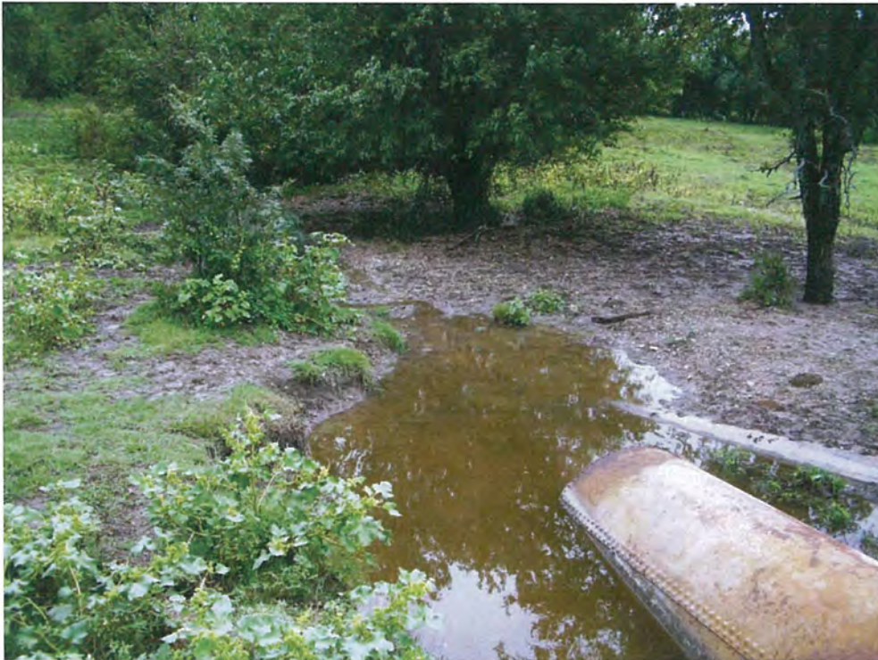
P13. Looking east (downstream) along LCT2. Stream has circumvented a culverted ranch road crossing in this location.
