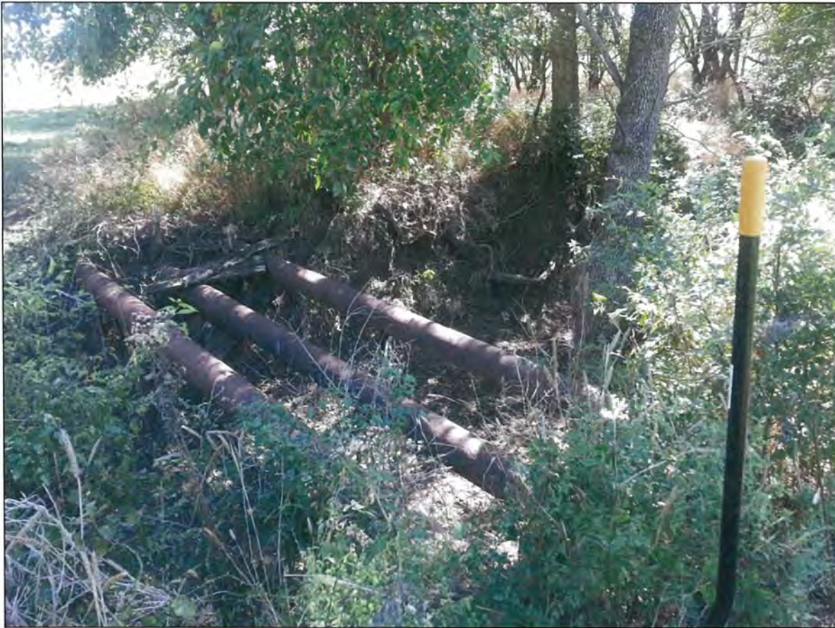
Figure 10. The survey corridor crossing of Ward Creek. The pipeline will cross near existing pipes.
