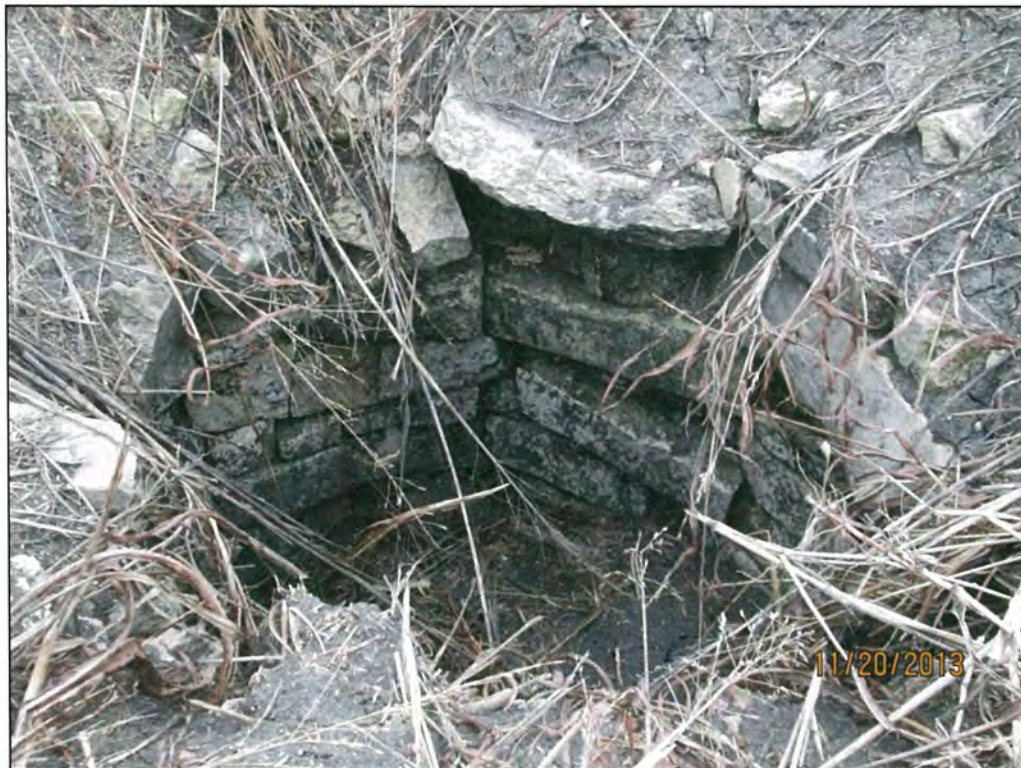
Figure 61. Close up of well-cistern at 41NF173 with view of dry laid limestone and fill.
