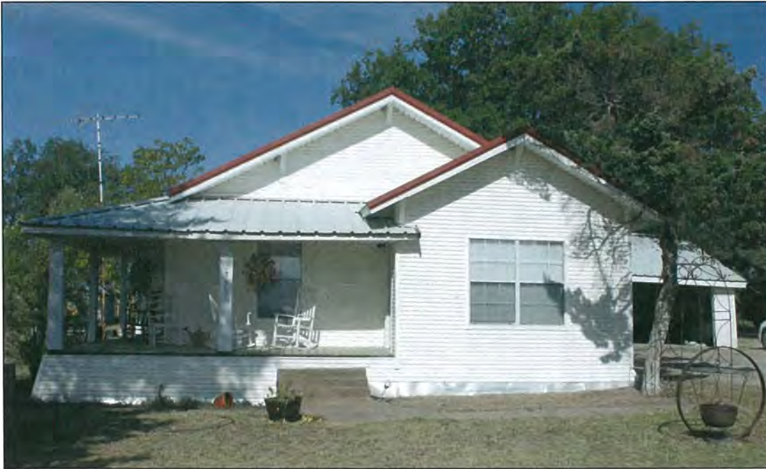
Figure 70. Resource 1a: Facade, looking west.
