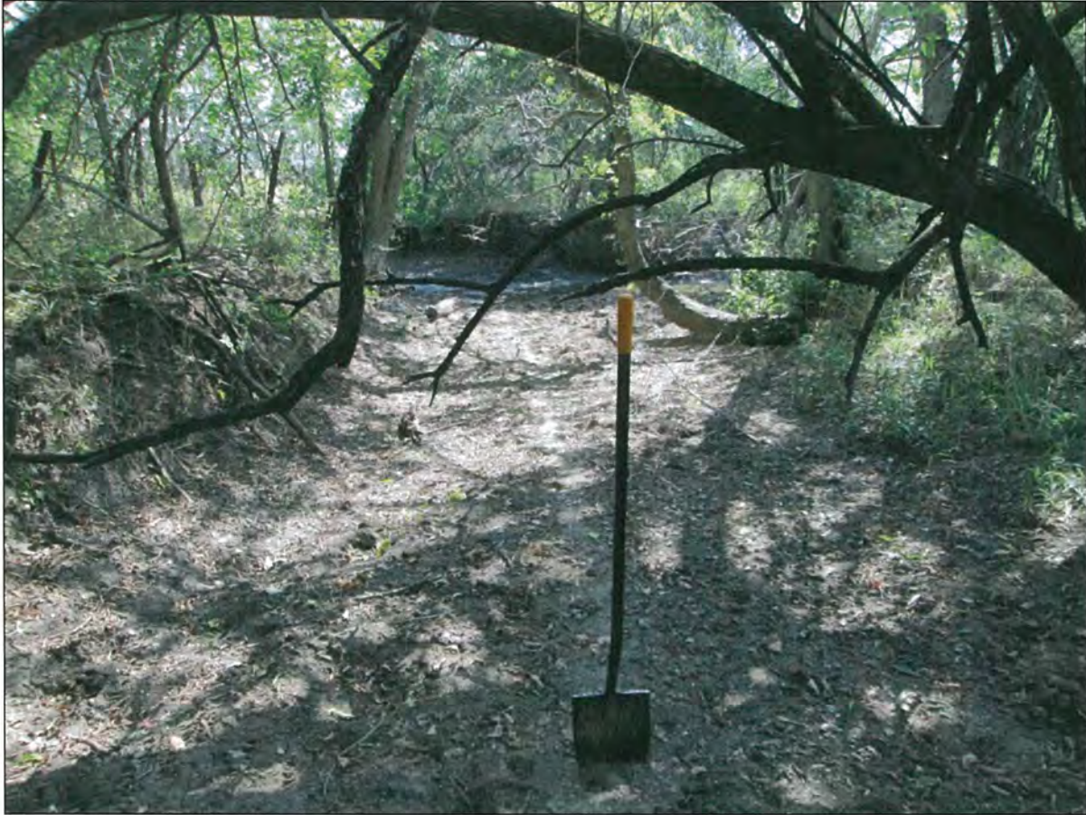
Figure 30. The proposed crossing of Lee Creek. Note the exposed bedrock in the background.
