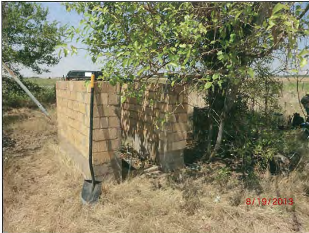
Figure 45. View of pump house opening; looking northwest.
