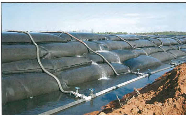
Figure 5: Geotubes (courtesy of TenCate)
