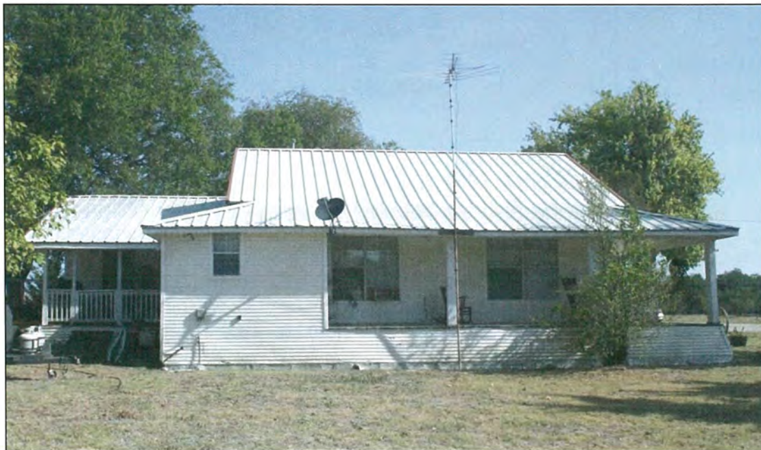
Figure 72. Resource 1a: South elevation, looking north.
