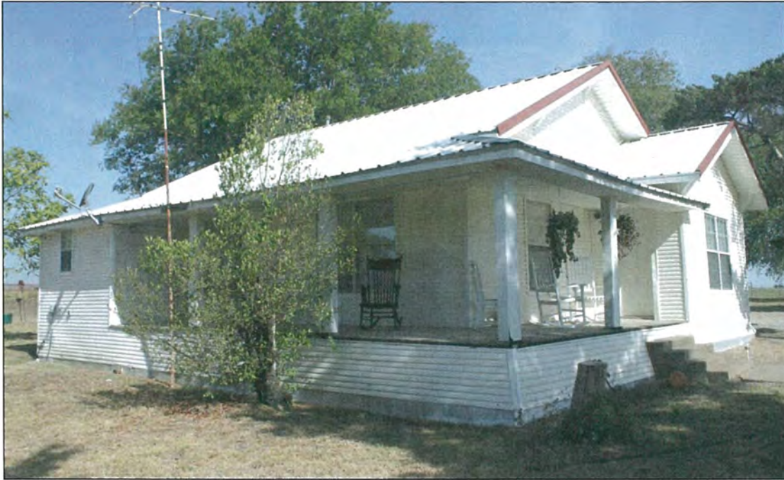
Figure 73. Resource 1a: Oblique of facade and south elevation, looking northwest.
