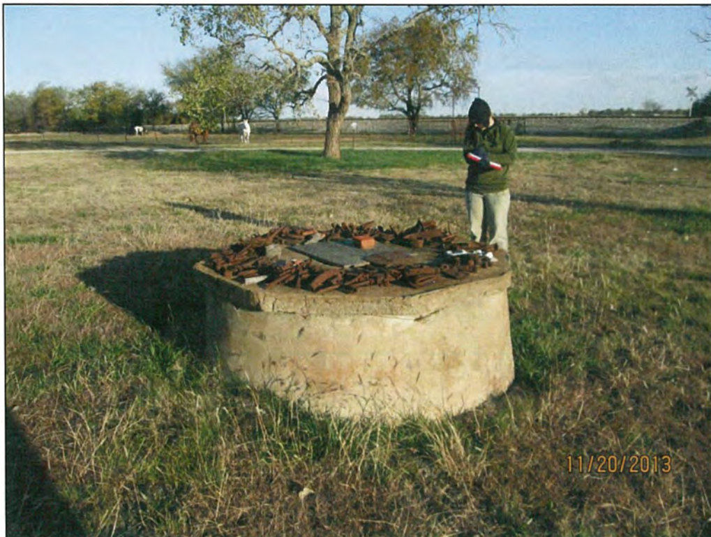
Figure 57. Well-cistern at 41FN172; view is to the north.
