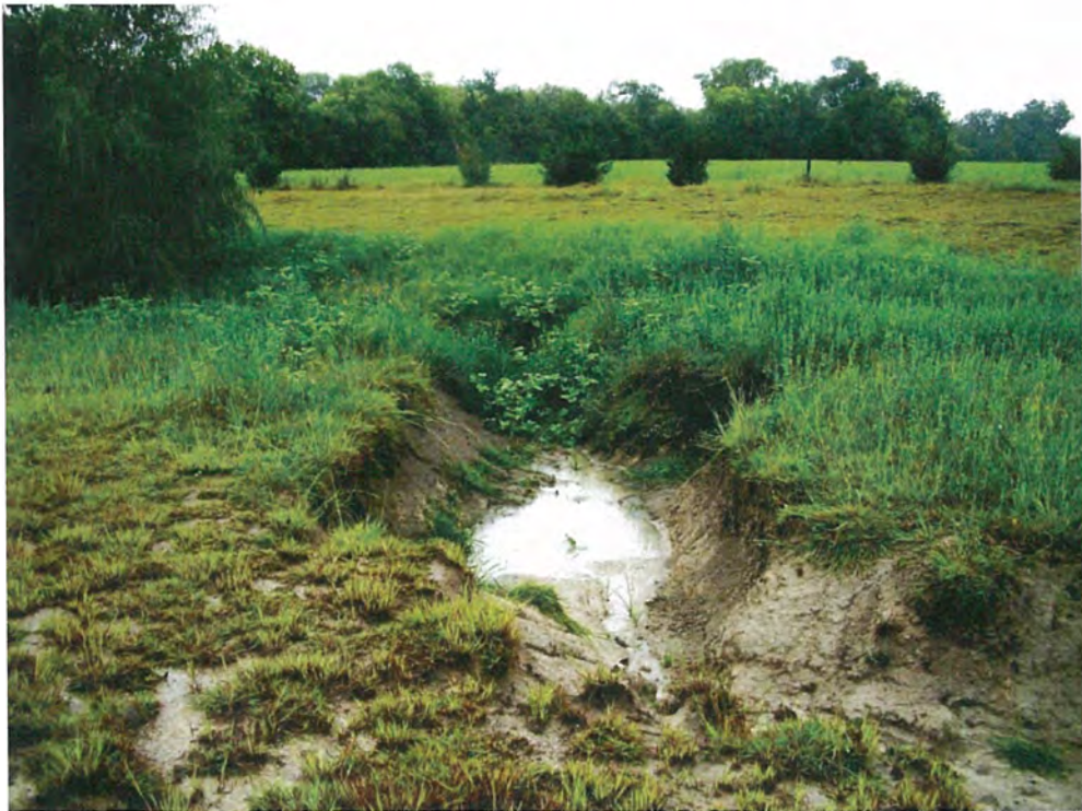
P48. Looking southwest (downstream) along TBCT1 near the breach in WI1.
