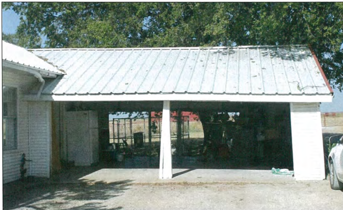
Figure 74. Resource 1a: Garage, looking west.
