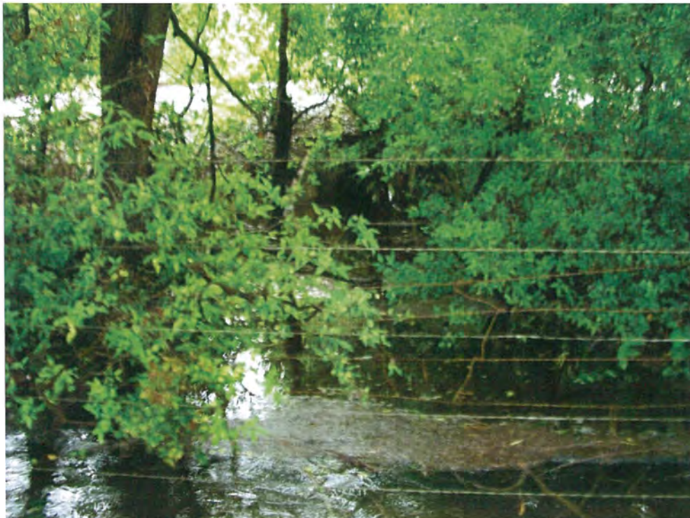
P20. Looking northeast (upstream) at LCT4 and EW1 where LCT4 enters the subject property beneath the MKT railro. (background of photograph).
