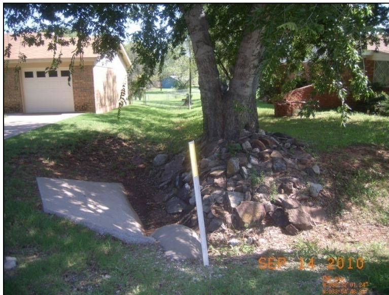
Photo 2 – Culvert outfall and channel on Wyneth Drive.
