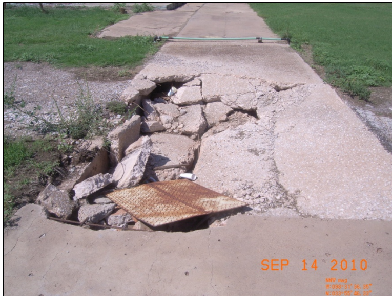
Photo 2 – East Plum Creek culvert located on 2812 Iowa Park Road.
