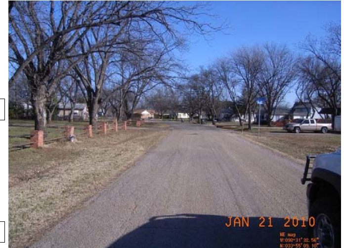
Wichita Gardens typical street section with no curb and gutter and very shallow road side swales.
