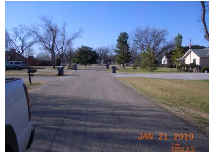
Homes at street level with no road drainage.
