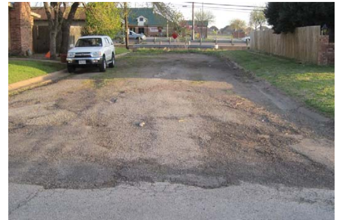
Looking south from Covington Drive at alley outfall into McGrath Creek.
