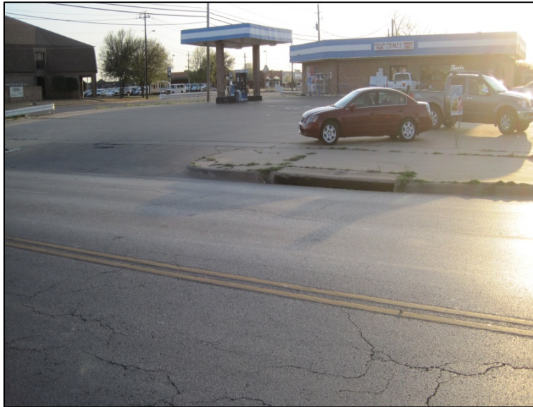
Photo 2 - Existing inlet on Rhea Road
