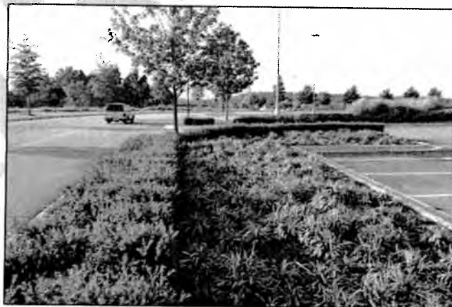
Figure 1.3.2-26 Parking Lot Storm Water “Island”
