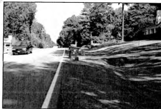
Figure 1.3.2-30 Using Vegetated Swales Instead of Curb and Gutter
