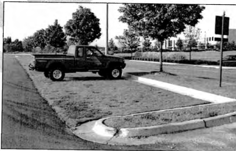
Figure 1.3.2-21 Grass Paver Surface Used for Parking
