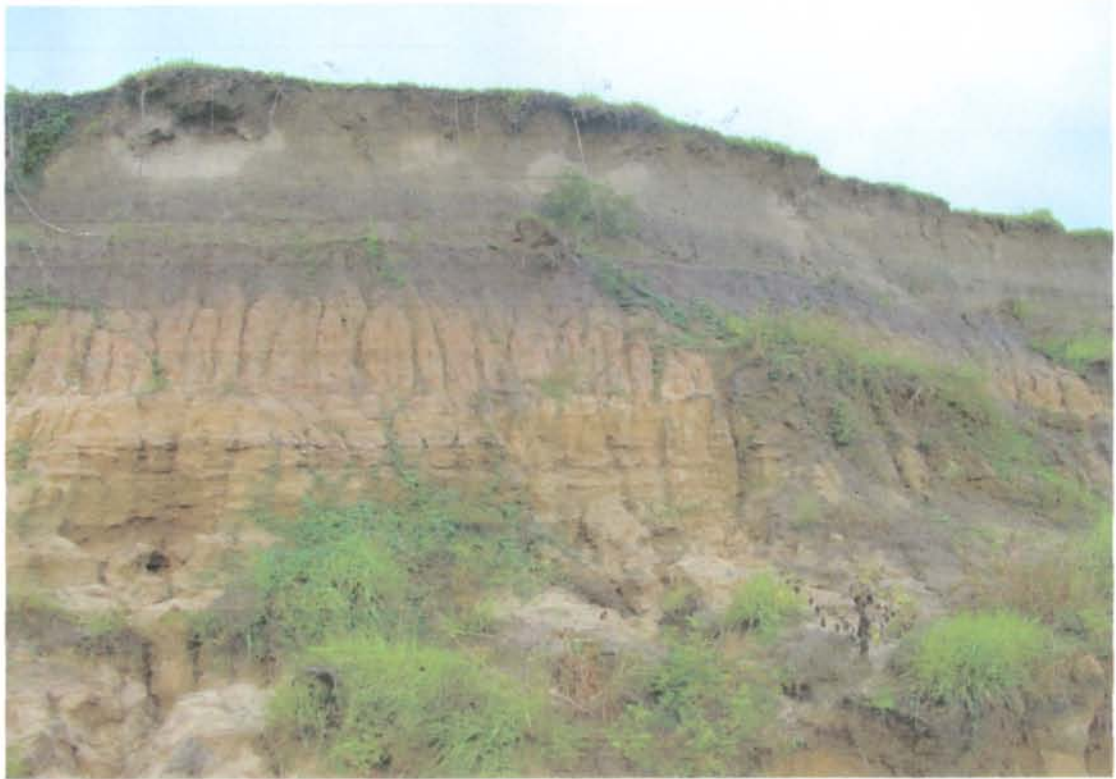
Figure 10. Channel bank erosion upstream of the gaging station at Romayor.
