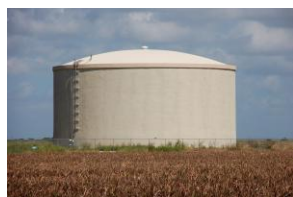
Construction of the ground storage tank, North Cameron Regional Water Project, March 2005.
