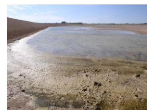
View of the evaporation pond for the City of Brady desalination facility. Water from the Brady reservoir is desalted and blended with well water from the Hickory aquifer. Concentrate is diverted into this pond, constructed in 2005, for evaporation.
