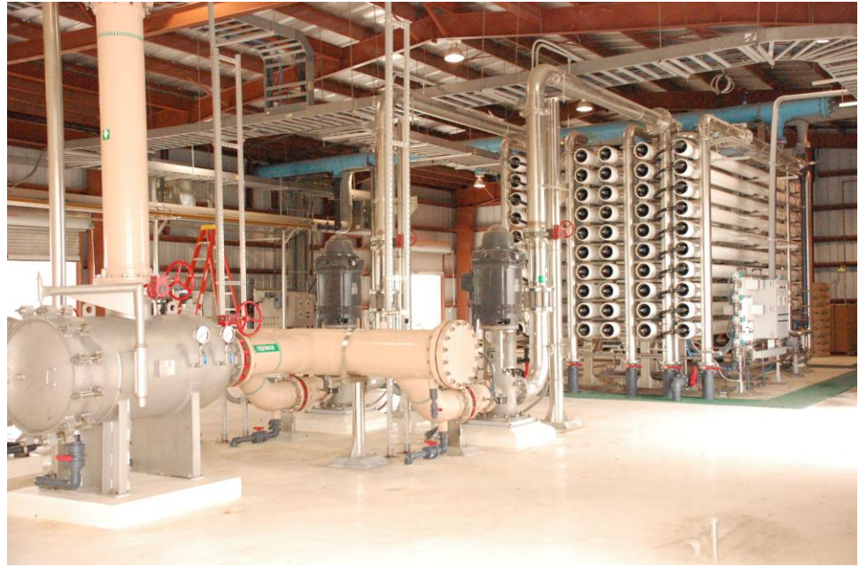
Key water treatment equipment, North Cameron Regional Water Project, August 2007. Photograph shows cartridge filters (left), stainless steel high pressure pumps (center) and reverse osmosis modules (right).
