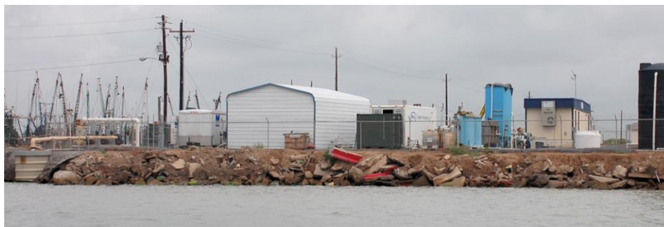
The Brownsville Seawater Desalination Pilot Project. Photograph courtesy of WaterPR
