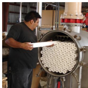
Installation of cartridge filters, North Cameron Regional Water Project, November 2006.
