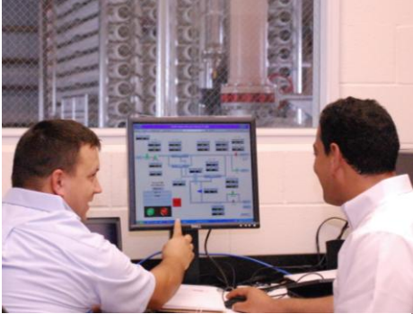
Training for the master control system, North Cameron Regional Water Project, June 2007.
