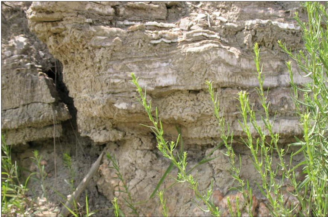
Gypsum bed in outcrop located at approximately 1/4 mile Northwest of proposed dam alignment
