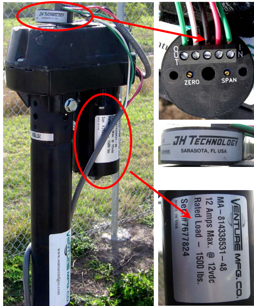
Figure 11. Gate actuator showing arm and motor (left), actuator arm position sensor (4-20 ma potentiometer) (Top right) and details of motor (bottom right).
