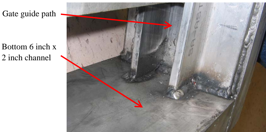
Figure 8. Construction of bottom of gate frame.
