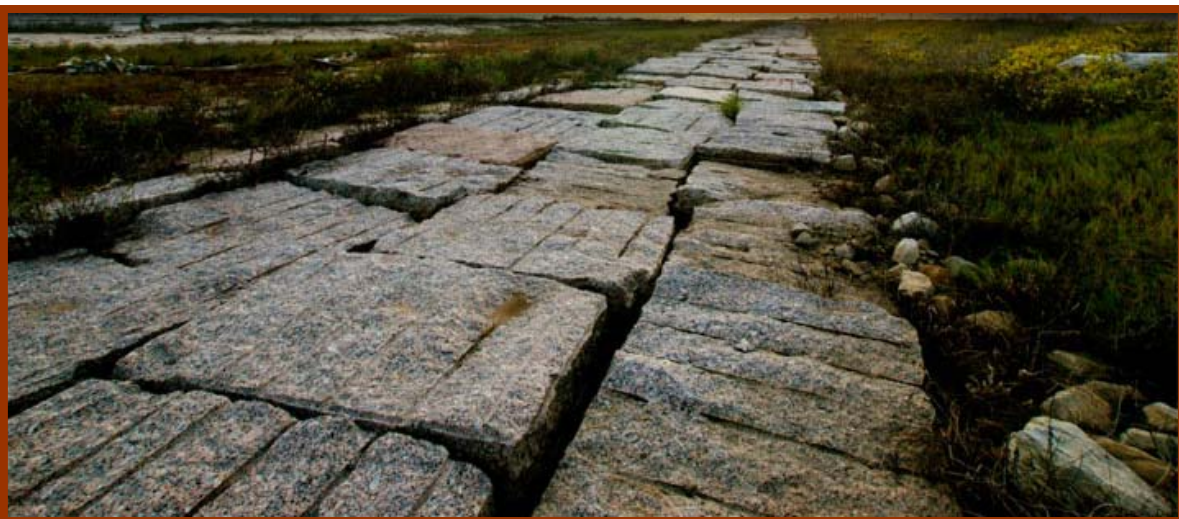
Figure 34: 8-Mile Sargent Beach Granite Revetment Wall
