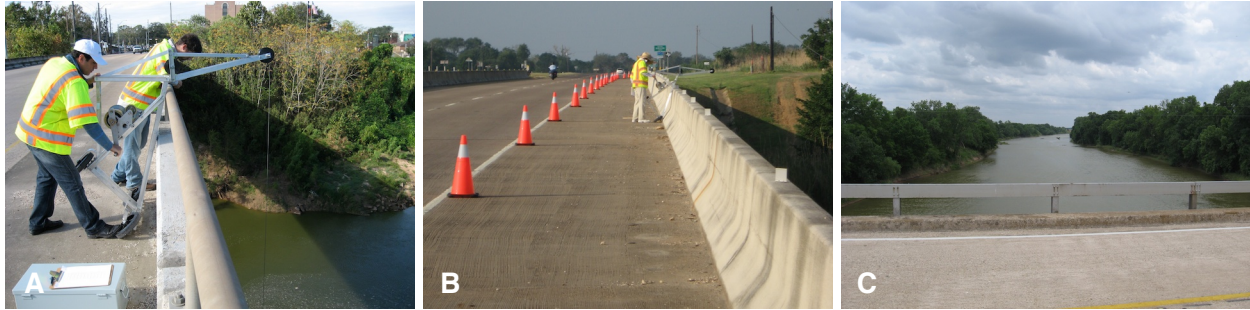
Figure 3.2: Examples of different shoulder conditions across the bridge deck. (A) the Richmond bridge with a pedestrian walkway; (B) the Bryan bridge with a shoulder closure; and (C) the Highbank bridge with no shoulder.
