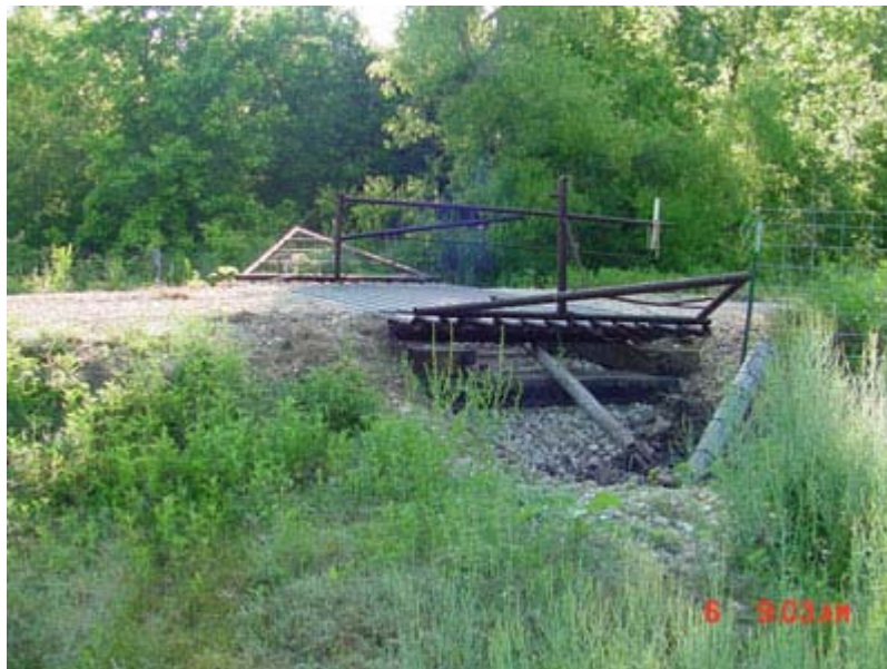
Figure 3.3 – Rectangular flow channel serves as control point for Moelhman Slough connections with the Brazos River.
