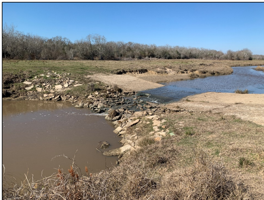
Figure 17. Barrier to flow on Big Boggy Creek. This structure (barrier 1 in Table 2 & Figure 16) does not appear to have culverts and instead allows the water to flow over the top.
